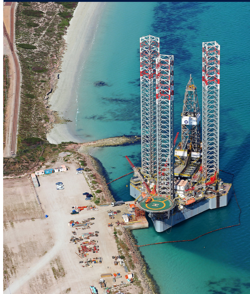
Figure 4: Port of Saldanha Bay
